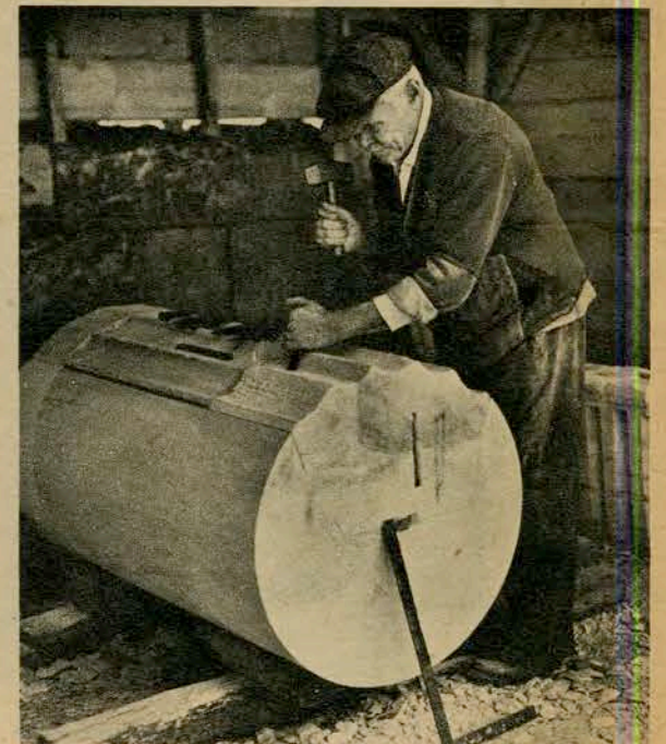
PILLAR: Cutter sets new marble into old by hand
