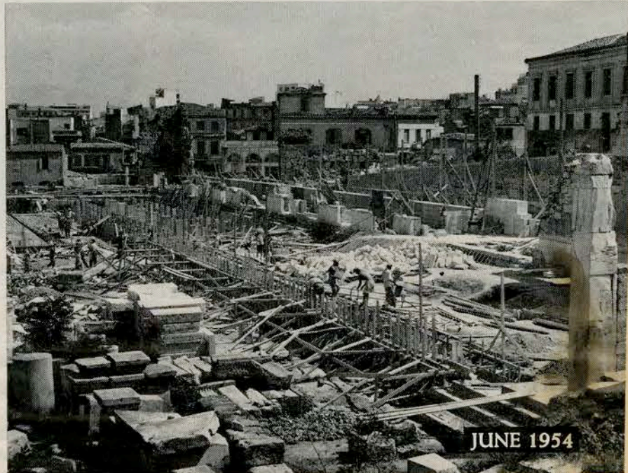
AFTER THE FOUNDATIONS WERE REINFORCED, FRONT STEPS WERE LAID
