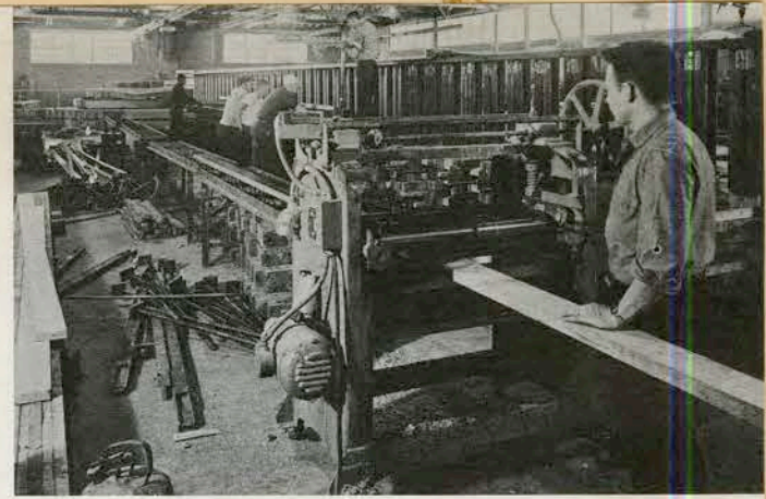
A UNIFORM COATING of glue is given to each ply of West Coast Douglas fir at the Rilco plant.
