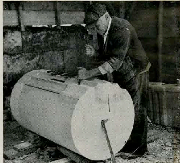
ANCIENT FLUTING, fragment of an original column, is fitted into new pillar. Sample pieces of all decorative motifs were set into rebuilt stoa.
