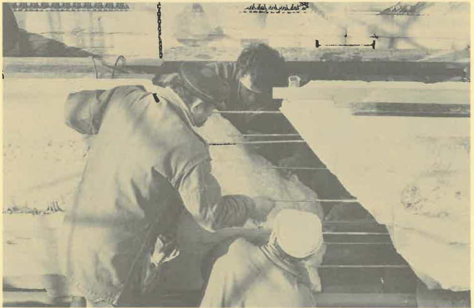
Two sections of architrave block are joined with titanium rods
