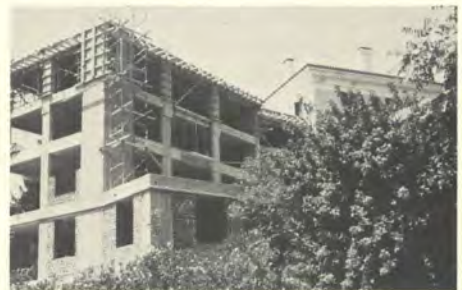
View from Gennadius Street: brick by brick, work on the extension to the Blegen Library proceeds on schedule. Photographed in mid-August, the addition has been topped off, and construction of walls has begun. The Main Building, which was repainted in late Spring, is visible to the right.
