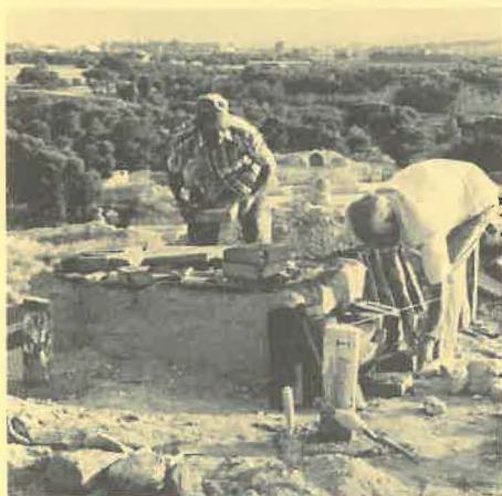
A kiln of sun-dried bricks is constructed to fire the roof tile
