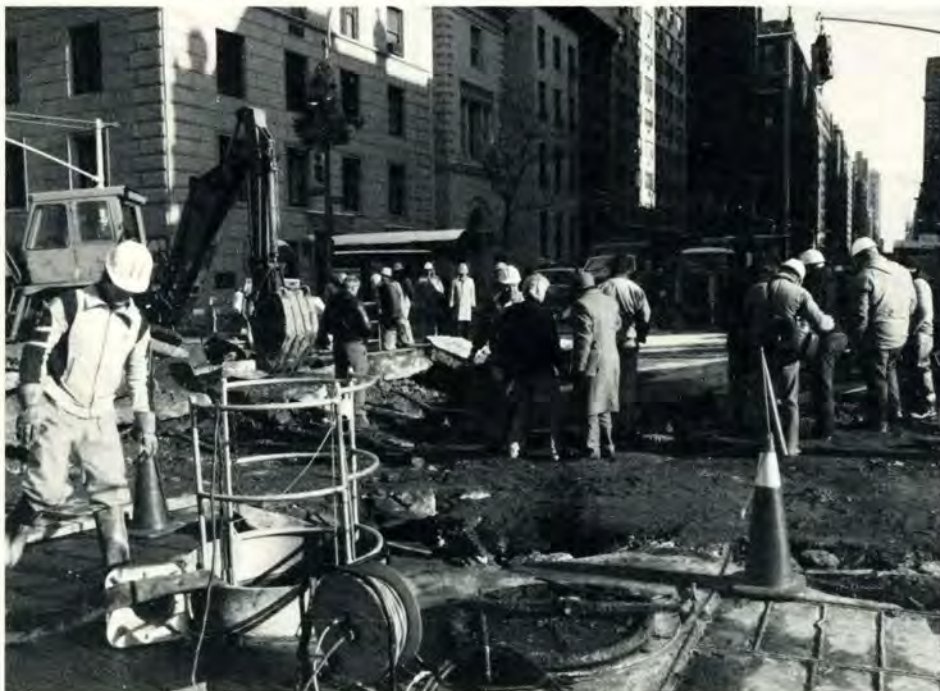
Scene inside and out: The basement of Mayer House, post-flood, and excavation at 72nd and Madison to repair the broken water mains.
