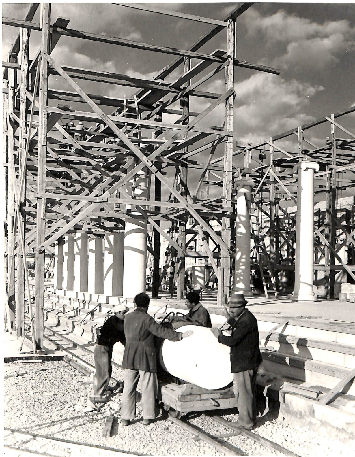
Scaffolding for setting up an outer colonnade. See Appendix 2, deposit # 13:1 (pp. 00-00)
