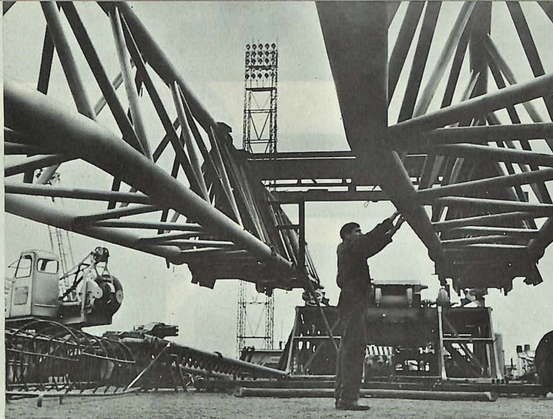
A full-view mast being raised into position
