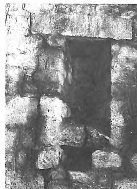
III. 6.—Wall slit, West gallery, with monolithic sill, broken later.
