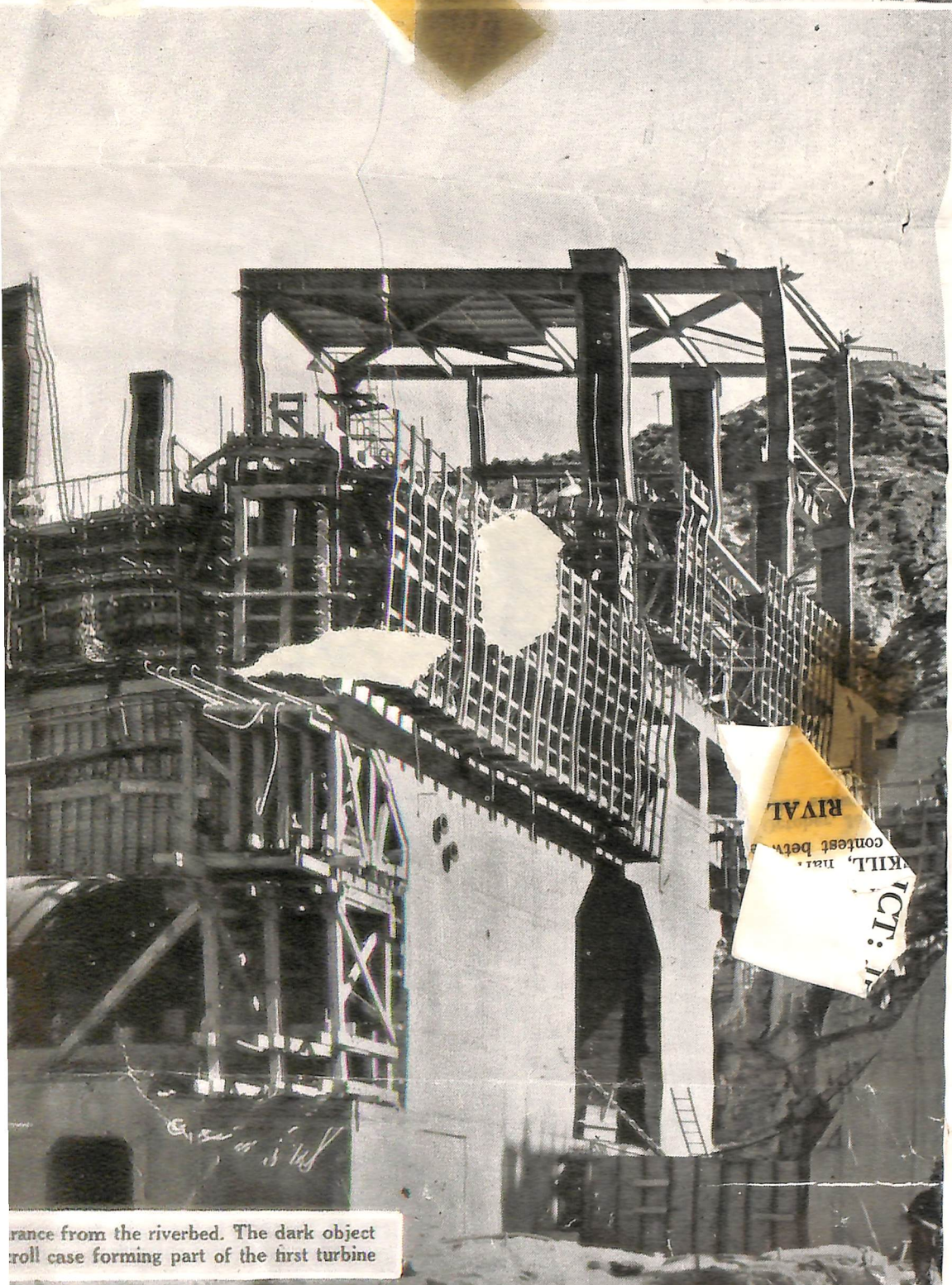
Looking from the old riverbed from the powerhouse construction to the dam. This has almost reached its full height. On the right are the head towers and on the left is the batching plant which is now working at full capacity.
