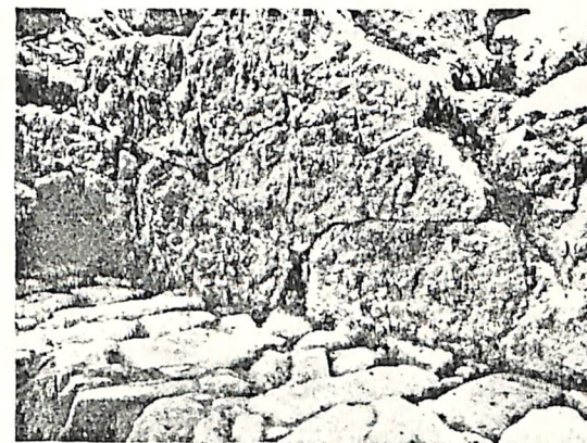
FIG. 4.—PAVING AND NORTH WALL.
